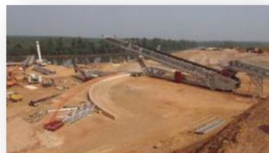
Mining project Marampa - Sierra Leone
