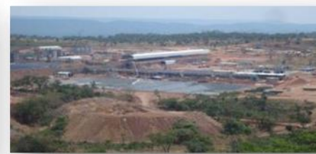
Mining project Tenke - DRC
